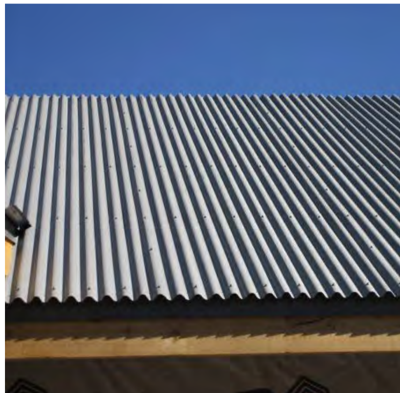
9 MR/XMRR, GALVANISED CORRUGATED ROOF Paint finish. Clear anti-graffiti coating.
