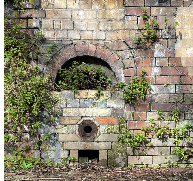
1 XBR, EXISTING BRICKWORK Repair, clean & repoint as required.
