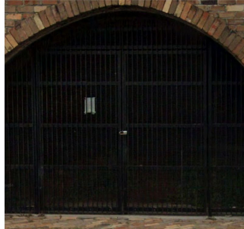
2 XMG, EXISTING METAL SCREEN AND GATE
