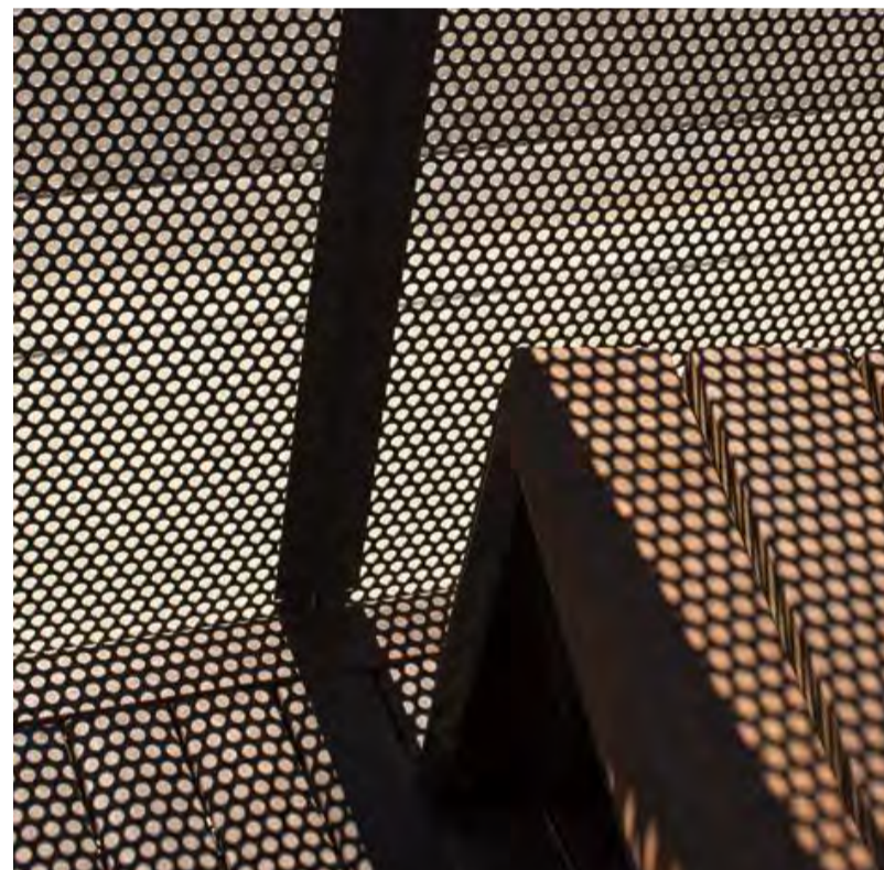
7 MCP, PERFORATED METAL SCREEN Approx. 50% open area. Paint finish. Colour similar to Colorbond 'Monument'.
